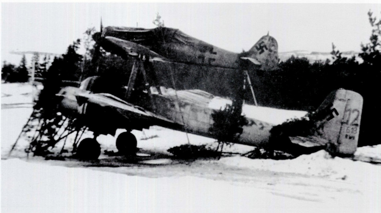
This photograph of an operational Mistel 2, 'Red 12', assigned to Fw. Rudi Riedl was taken in early 1945 at Tirstrup, Denmark. The Ju 88 G-1, W.Nr. 714050 has had the front cockpit section replaced with a hollow charge warhead, suggesting imminent operational use. Some primitive attempt has been made to camouflage the aircraft by parking them near some trees and using branches and tarpaulins to hide them from Allied reconnaissance. The 'RW' number 618 also painted in red on the rudder of the Ju 88 was the Reperaturwerkstatt (works conversion) number applied by the Junkers works at Nordhausen.
