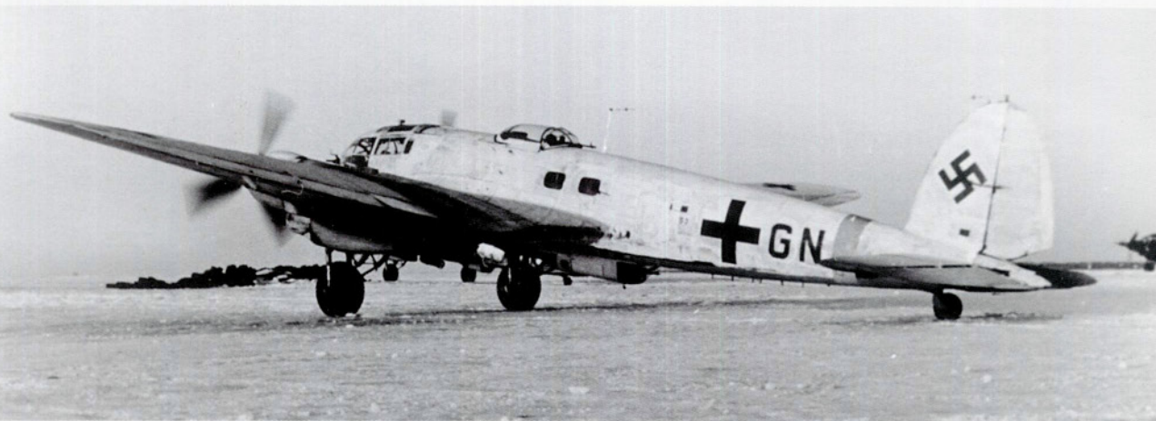
LEFT: This He 111 H-16 belonging to 5./KG 4 'General Wever' is coded 5J+GN, taxis to its take off point. The fuselage has been overpainted in temporary white winter paint but the wing upper surfaces have been left in the standard 70/71 camouflage. The Eastern Front yellow band has also been painted around the rear of the fuselage.
