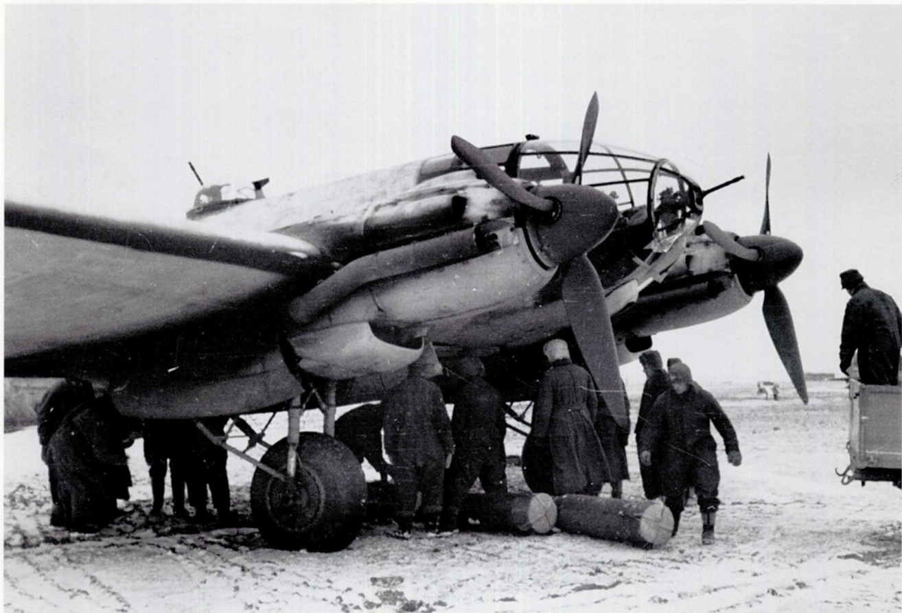
LEFT, BELOW AND OPPOSITE: By early 1945 many bomber aircraft were pressed into transports supplying bypassed troop pockets and cities where heavy fighting was still taking place. These aircraft were often simply overpainted with white winter camouflage paint, which obliterated the unit codes. These three photographs of a He 111 H-20 fitted with a towing hitch, is evidence of this practice.
